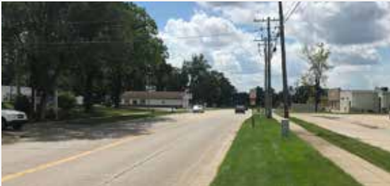
EXISTING CONDITIONS: ROBINS ROAD
